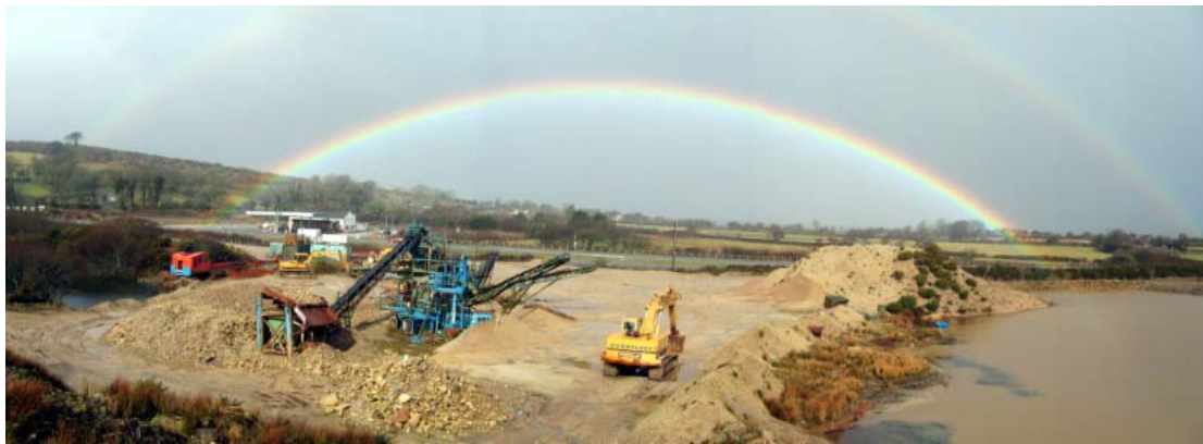
Sand and gravel recovery operation at Trewint
