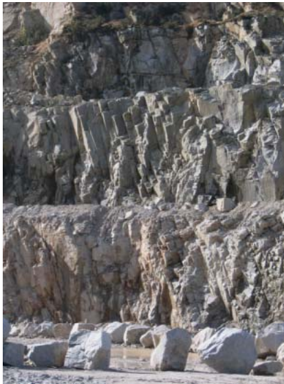
Sub-vertical joint set
