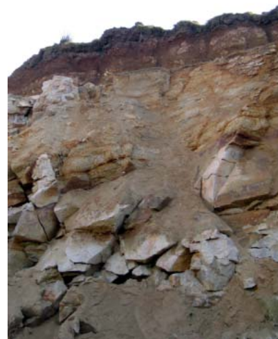
Weathering profile from soil, subsoil to bedrock
